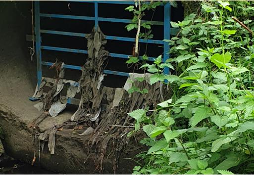
During heavy precipitation events, wastewater is often released directly into bodies of water to relieve the pressure on sewage treatment plants. Wet wipes, sanitary pads and tampons, among other things, get swept along with the wastewater and pollute the environment.
